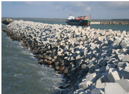
Figure 47: Photo of fortified breakwater off marina.
